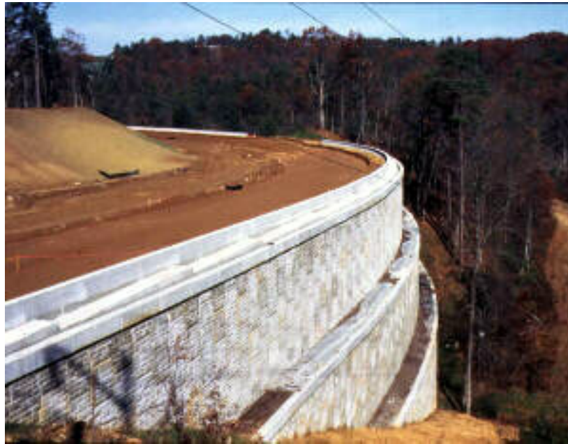
Exhibit 3-51: Double Track Retained Earth Fill
