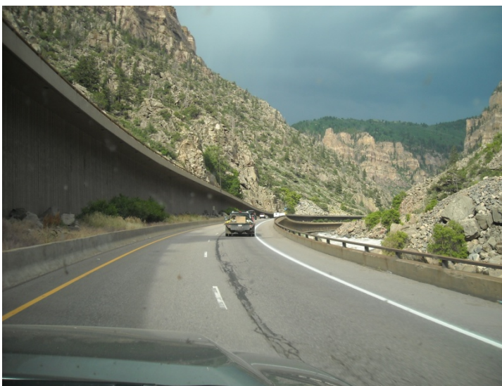
Exhibit 3-46: View east along the I-70 corridor (MP 124) through Glenwood Canyon
