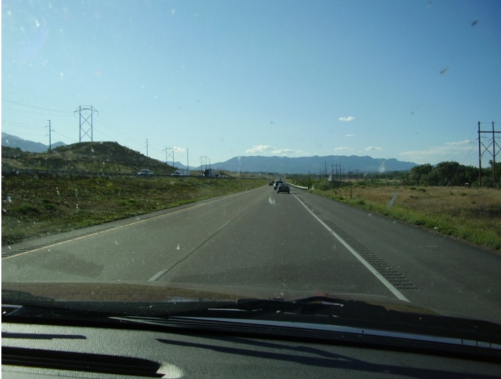
Exhibit 3-10: I-25 at MP 125 South of Colorado Springs, View North
