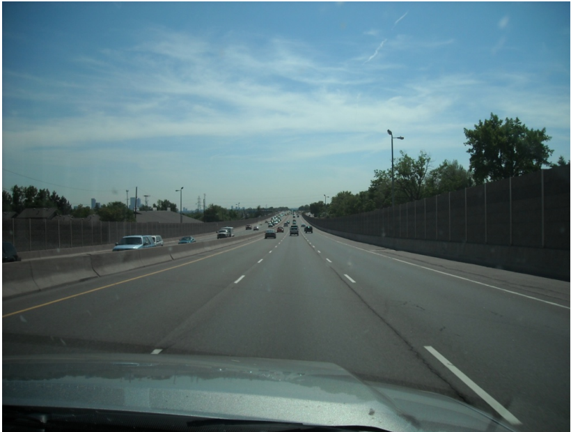
Exhibit 3-33: US-6 near Denver city limits in a very constrained area
