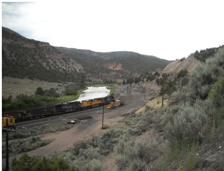
Exhibit 3-47: View west toward Dotsero along the UPRR
