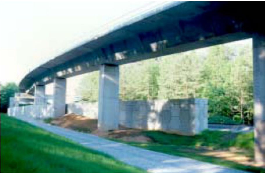
Source: Reinforced Earth Company
