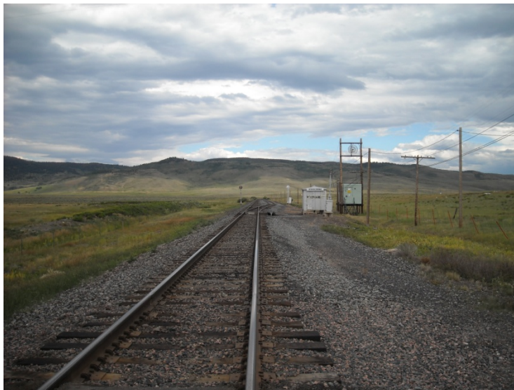
Exhibit 3-48: View south on the UP Branch line to Bond at CP 153 near Toponas
