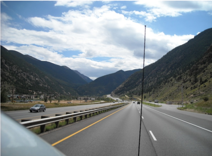
Exhibit 3-38: View west in the vicinity of MP 230 approaching Georgetown
