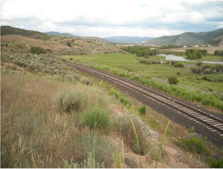
Exhibit 3-44: Typical View of condition of UPRR Tennessee Pass Subdivision
